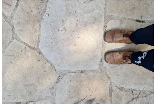
Stone paving that was designed for accessibility for the Nahal HaShofet project: a bush hammered stone, processed to look natural, with minimal force at the height of the stone to get most of the surface leveled and without protrusions Photo: Bella Nudelman
